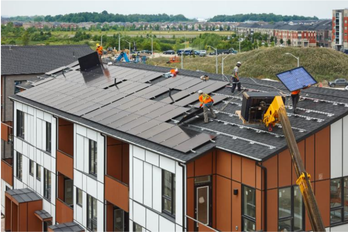
Installation of the solar panels
