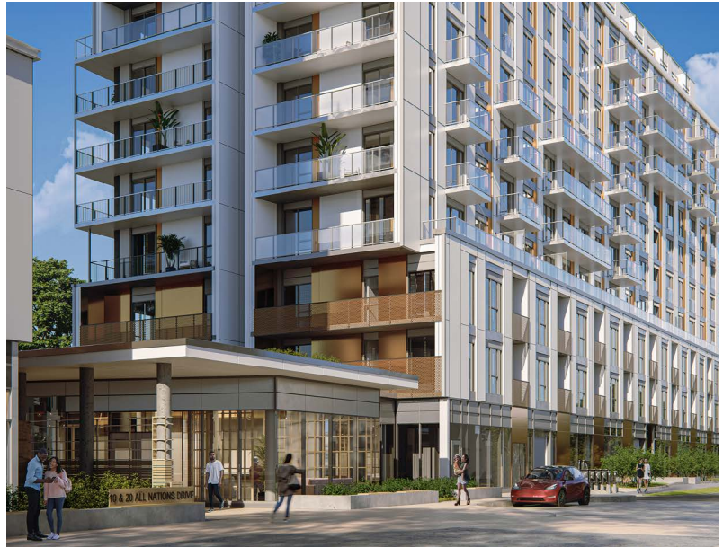
Figure 13.1 – Daniels MPV2 Condominiums, Brampton, Sidewalk View
