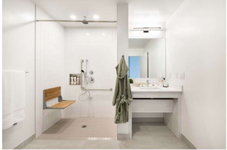
Figure 5.3 - Example Photo of ADP Accessible Bathroom
